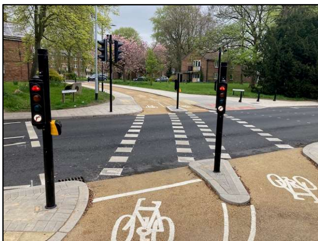
First completed Cyclops junction in Hulme, Manchester.
